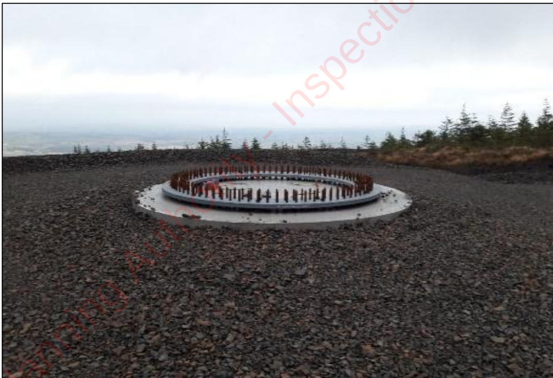
Plate 4-3 Finished Turbine Base
