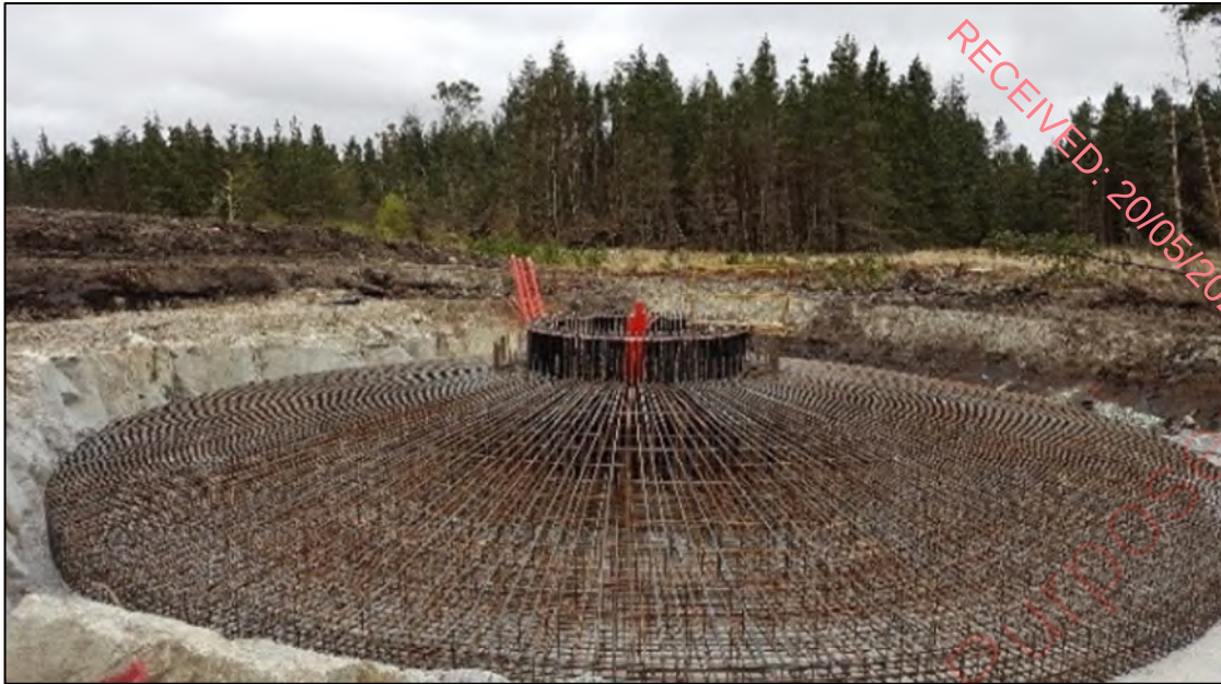
Plate 4-2 Turbine Base Anchor Cage surrounded by reinforcing steel.
