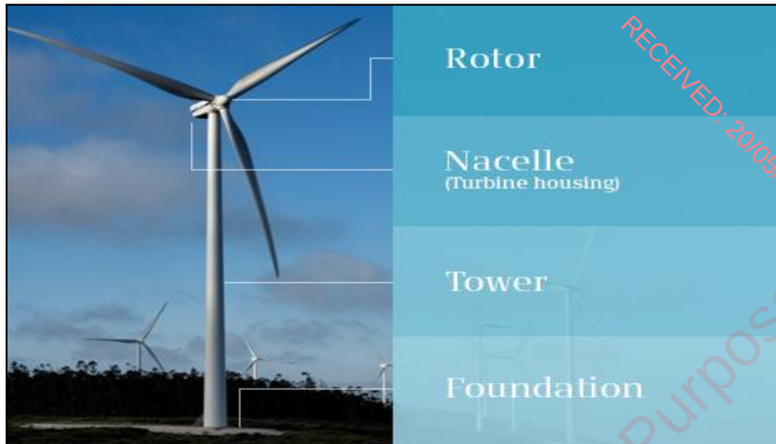
Plate 4-1 Wind Turbine Components
